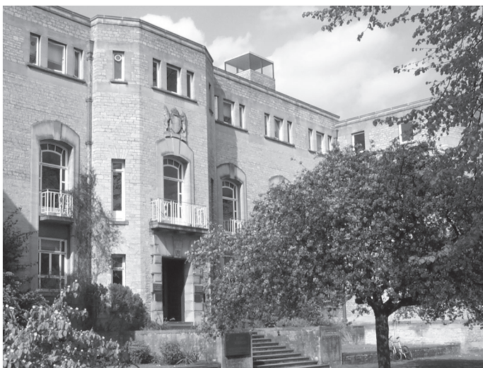
Figure 2 Plant Sciences (Forestry) building - library on first floor
