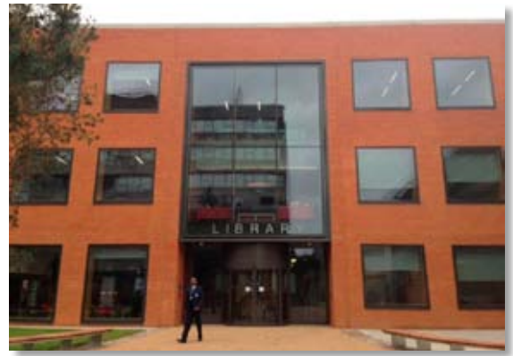
The new Stratford Campus Library
